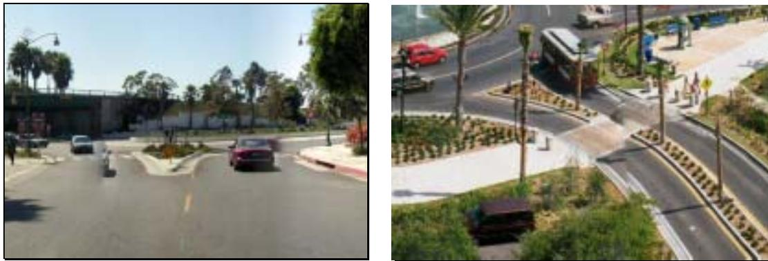
Figure 50 Median splitter islands and set-back crosswalks create safe pedestrian crossings
