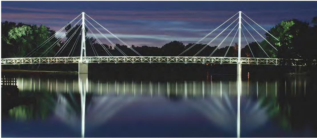
Figure 11. Example of a cable-stayed bridge
