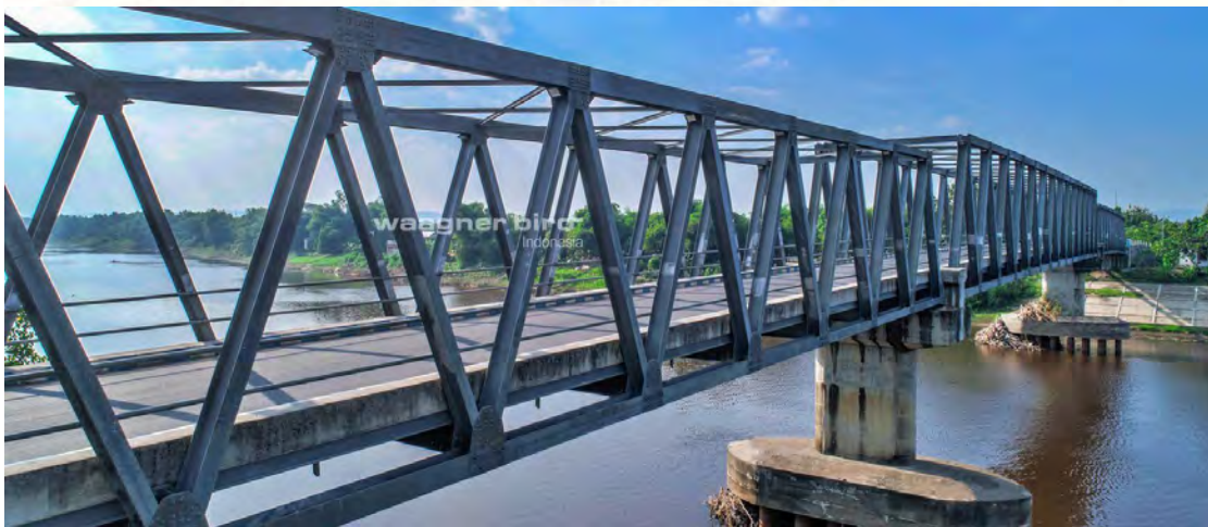
Figure 12. Example of a standard truss bridge
