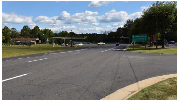
A Continuous Green-T (CGT) intersection improvement is proposed in SMART SCALE Round 5 for the current four-way signalized intersection at Routes 3 and 20 in Locust Grove.
