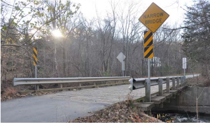
Route 638 bridge over South River
