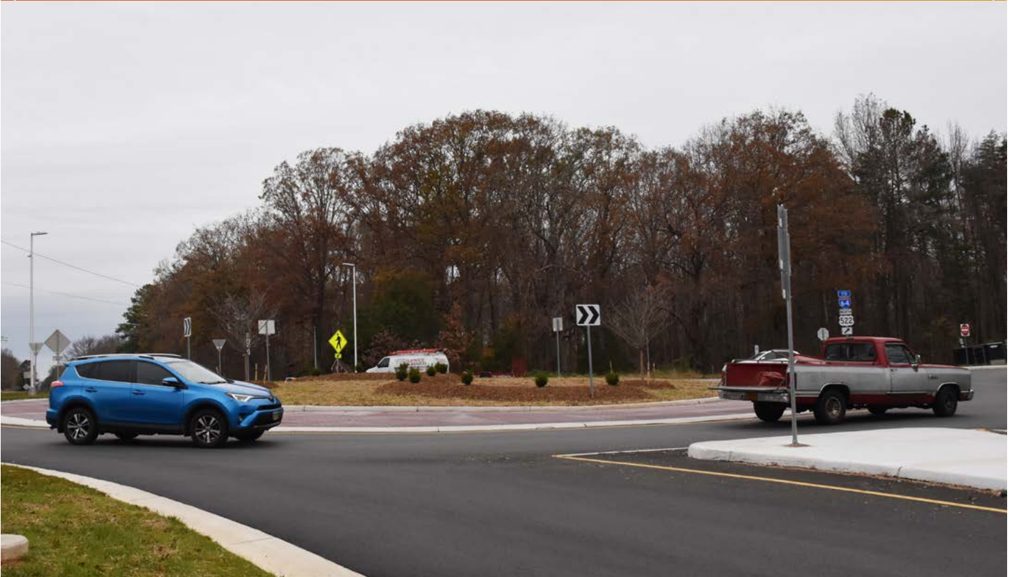
Construction of the roundabout at U.S. 250 and U.S. 522 in Gum Spring was completed in August.
