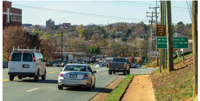
Two SMART SCALE projects are being bundled to reconstruct a segment of U.S. 250 (Richmond Road) between Route 20 (Stony Point Road) and Rolkin Road at Pantops.
