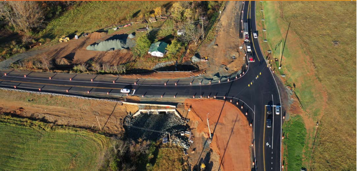
The roundabout at U.S. 250 and Route 151 at Afton is entering the final phase of construction, with traffic switched to the final configuration in mid-November.
