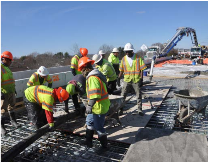
Crews pour concrete for the new deck of the U.S. 17 Southbound bridge over Norfolk Southern Railroad and Route 805.
