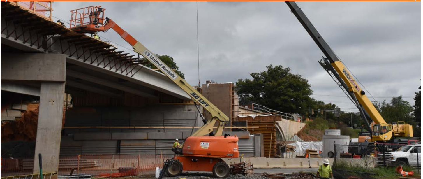
The aging Belmont Bridge in Charlottesville is being replaced through a $35.4 million project. Construction is under way; completion is scheduled by January 2024.
