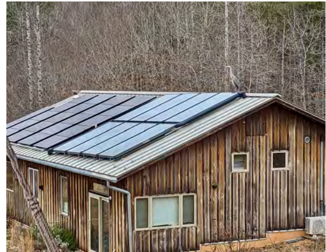
Solar panels on the roof of a resident's home in the Rural Area.
