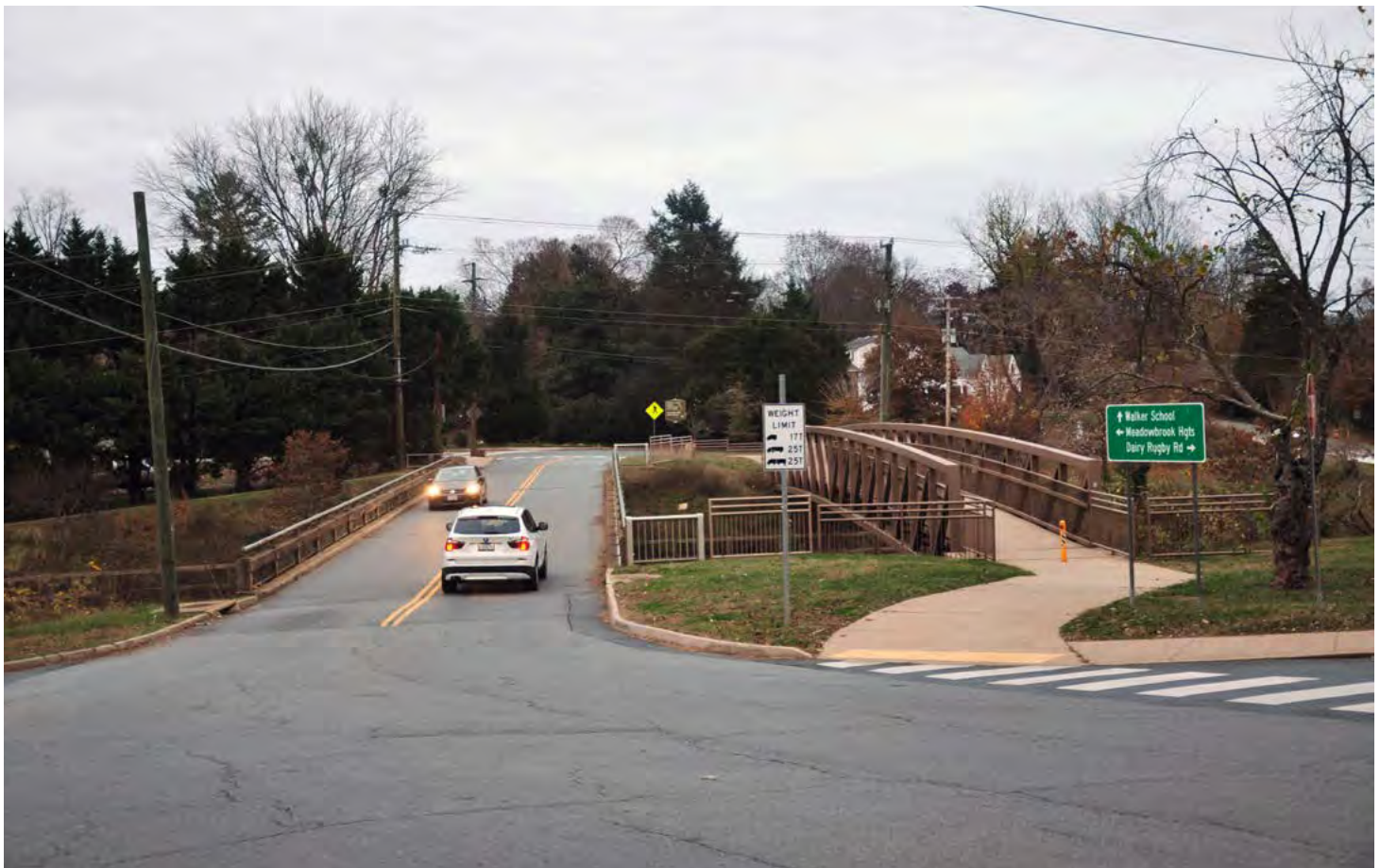
Preliminary engineering work continues on the locally administered project to replace the Dairy Road bridge over the U.S. 250 Bypass. To the right is the recently completed pedestrian bridge over the U.S. 250 Bypass.
