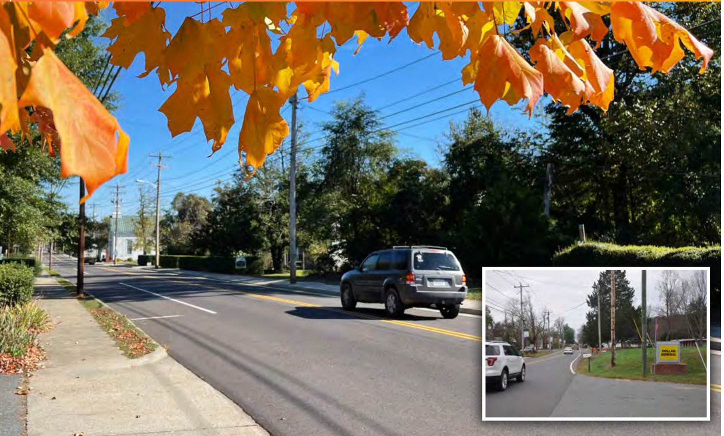
A sidewalk extension project on South Main Street in the town of Madison will enhance pedestrian access just as the color-changing leaves enhance the street's beauty each fall.
