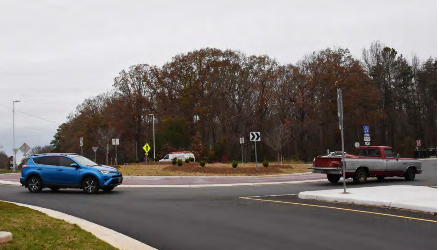
Construction of the roundabout at U.S. 250 and U.S. 522 in Gum Spring was completed in August.
