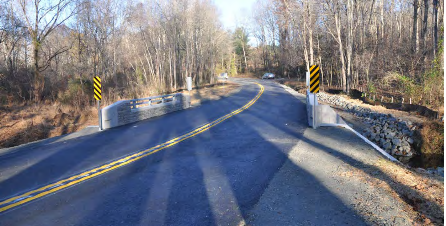
Replacement of the Route 647 bridge over the East Branch Thumb Run was completed Nov. 9.
