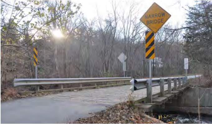
Route 638 bridge over South River
