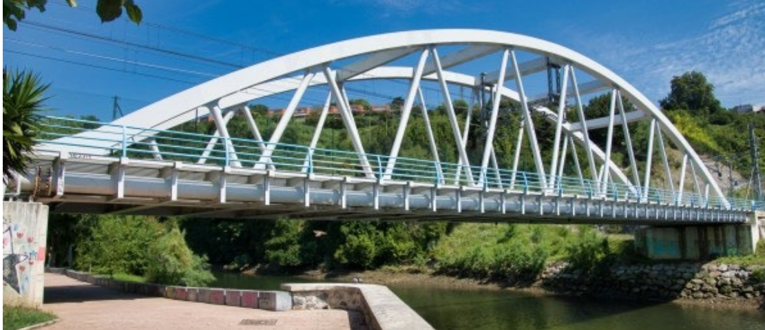
Figure 13. Example of an arched truss bridge
