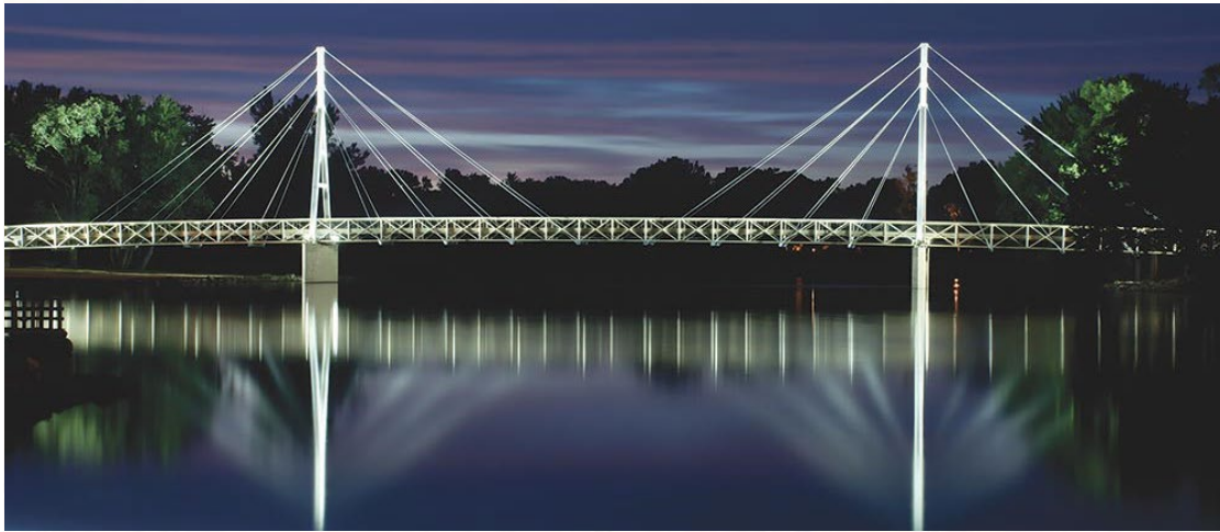
Figure 11. Example of a cable-stayed bridge
