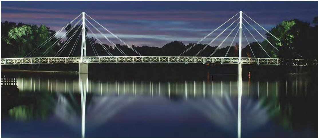
Figure 11. Example of a cable-stayed bridge
