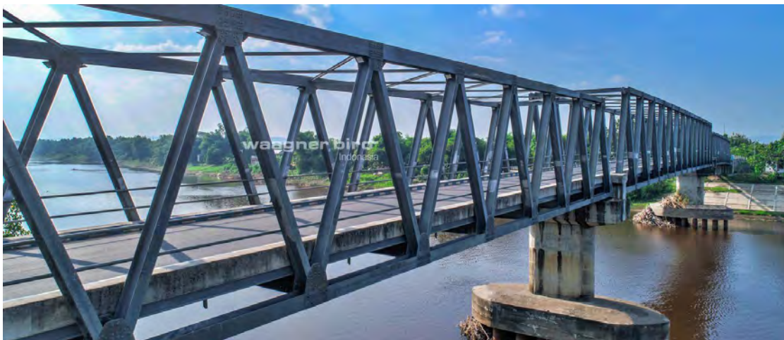
Figure 12. Example of a standard truss bridge
