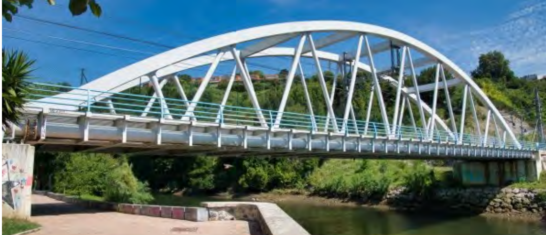
Figure 13. Example of an arched truss bridge
