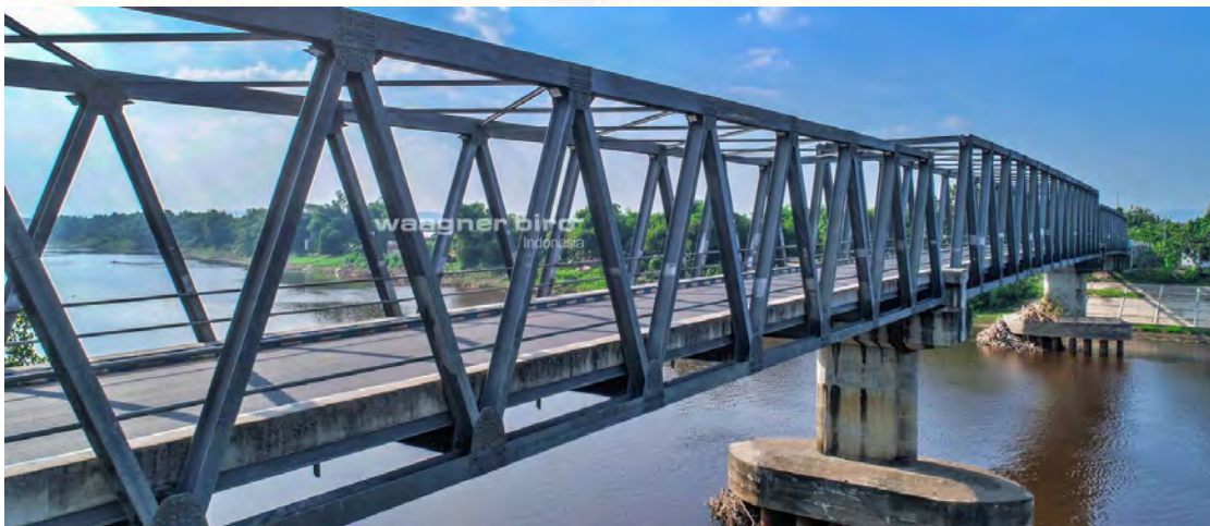
Figure 12. Example of a standard truss bridge
