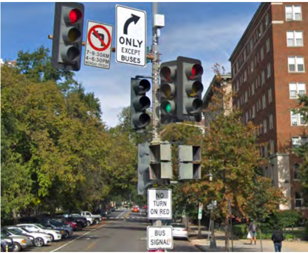
Figure 37: Dedicated signals and turn lanes are potential strategies to reduce delay for BRT vehicles.
